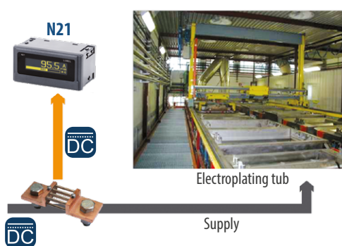
Current measurement in an electroplating plant
