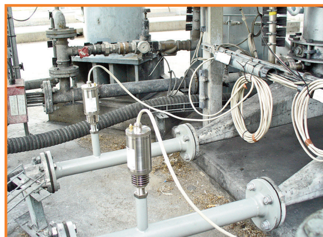
Mass flow measurement of calcium carbonate
